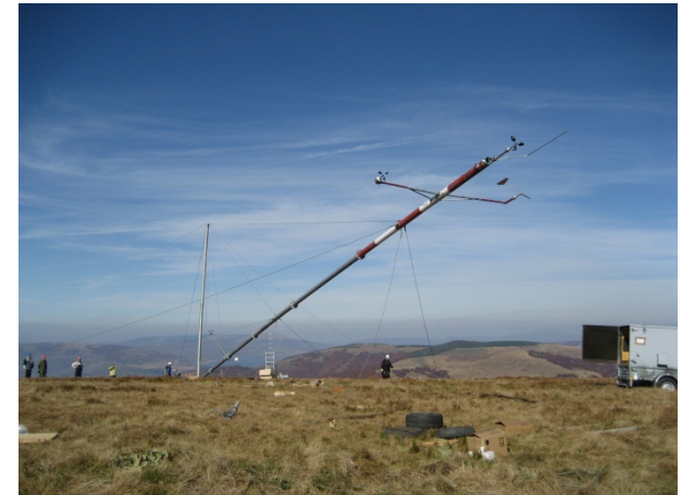
Photo: Installation of WM mast
