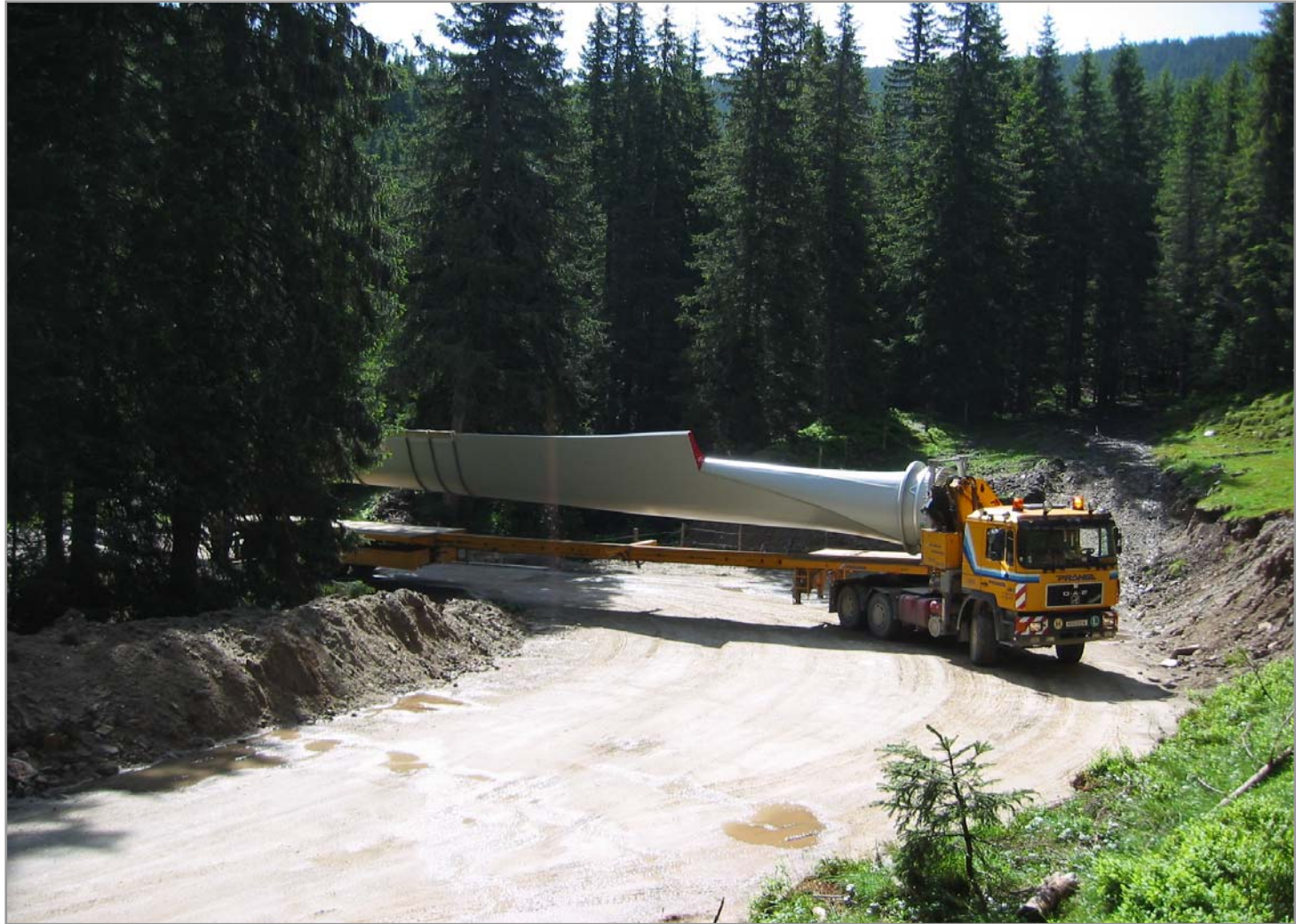
Construction of Wind Farm Moschkogel
